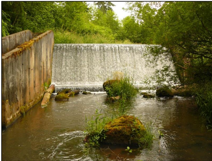
Figure 1. Odell Creek Hydroelectric Dam. The fish ladder is on the left side of the photo.
