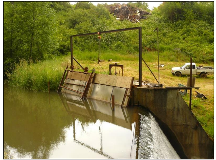
Figure 2. Existing fish screen
