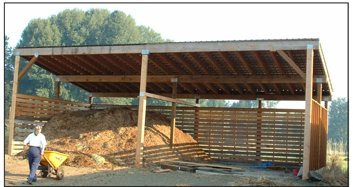
Covered manure storage facilities like this one protect nearby waterways from contamination while providing landowners with valuable compost for pastures.
